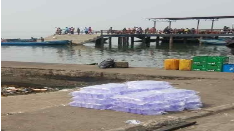
Plate 1: ATC jetty Okrika – a commercial jetty Source: Author's work (2021)
